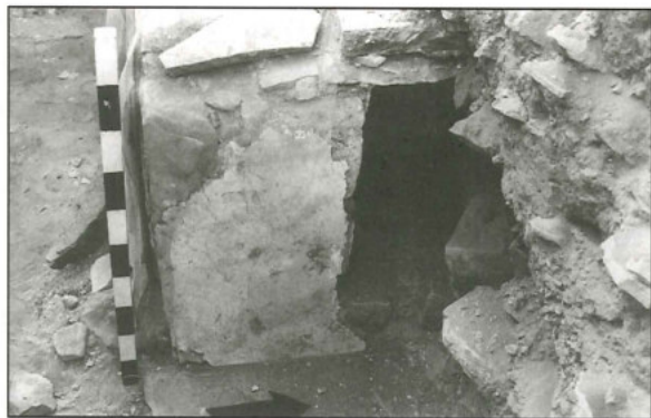
8. Trench C. The entrance to the compartment inside the masonry altar base (seen from E).
