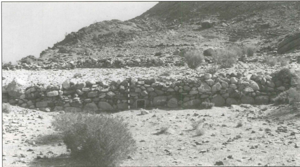
15. Tract 24, Site 33. Barrages built across the wadi.
