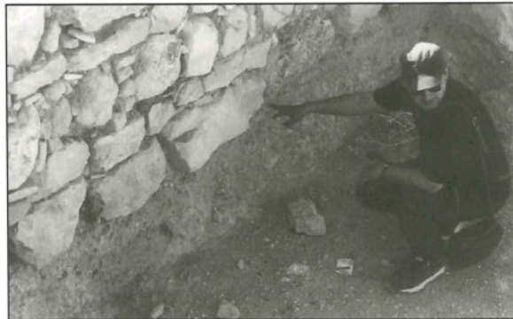
3. Foundation of the Late Islamic house on top of a foundation of compressed alluvial limestone gravel.
