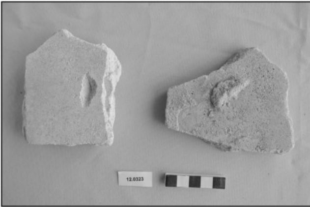
34. Top of an old layer of wall plaster punched (left) to key the underside of a new layer (right).
