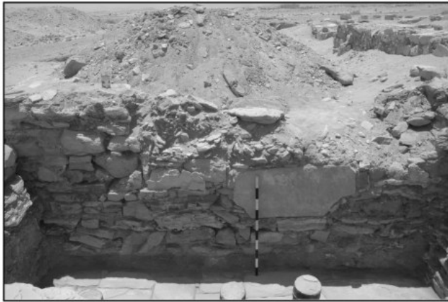
25. Praetorium Room J's south wall. Note the 19 cm thick layer of compacted sand located between the lowest course of wall stones and the top of the flagstone subfloor.
