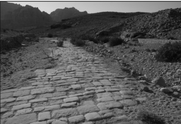
29. View of street east of the decumanus maximus (looking west). See Figure 1 (inset at top left). Photo by S.E. Sidebotham.
