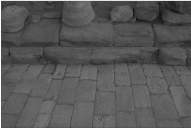
31. Damaged curbstones on southern side of decumanus maximus at its eastern end (looking south). Scale = 60 cm. Photo by S.E. Sidebotham.
