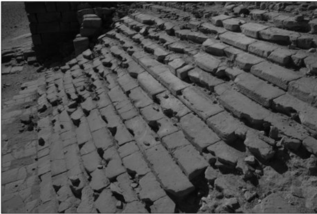
25. Staircase A at eastern end and on southern side of decumanus maximus (looking east). Photo by S.E. Sidebotham.
