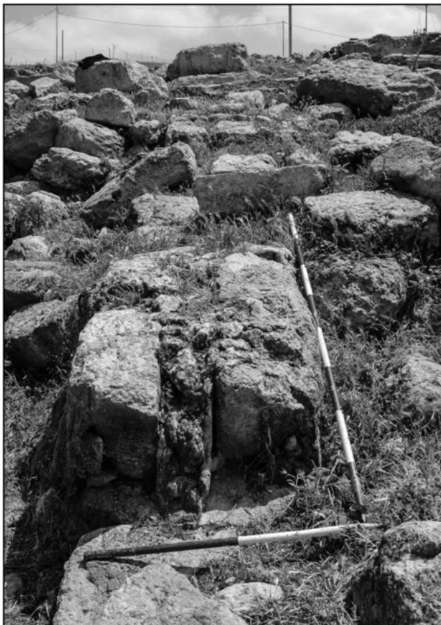
18. Masonry aqueduct below 'Ain Tannur (site 135). The specus is entirely filled with carbonate sediment.
