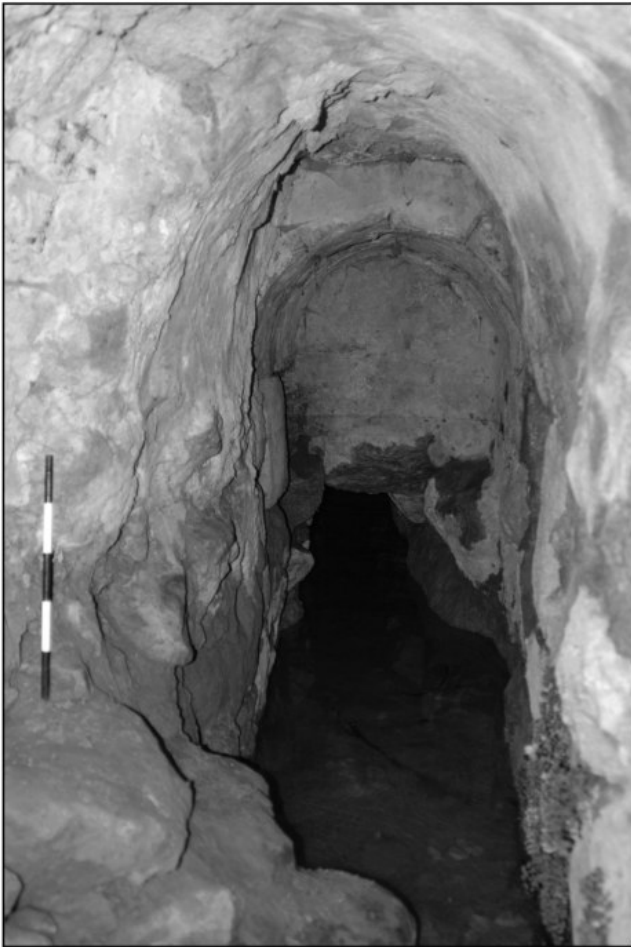
8. View of spring tunnel with corbelled roof at Muqibleh (D. Boyer).
