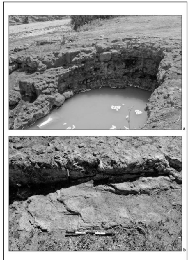
19. (a) Roman concrete foundations surrounding el-Hammām mineral spring (site 108) (D. Boyer). (b) Ancient concrete, faced with structura testacea , on west side of structure (D. Boyer).
