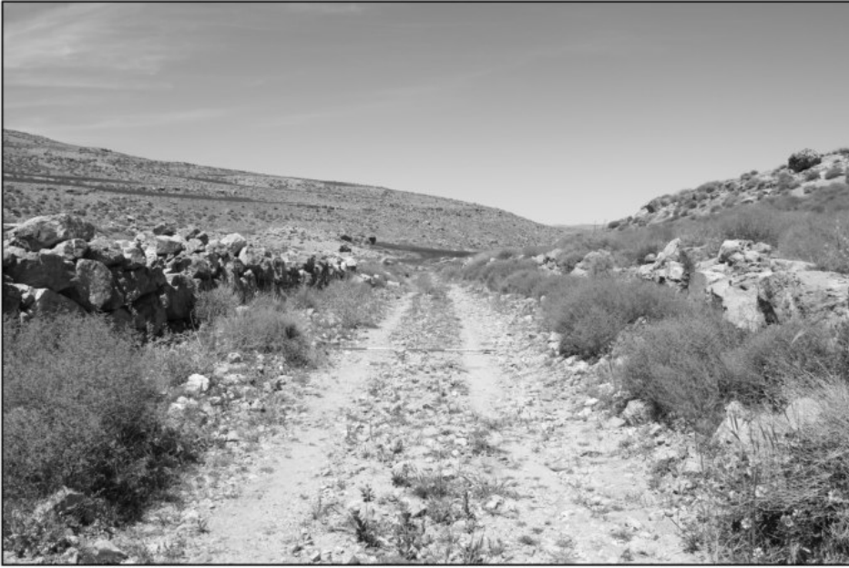
4. Photo of two retaining walls defining the path of the Via Nova Traiana south-east of Petra (© F. Abudanah).
