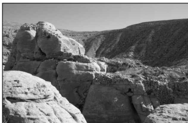
23. Overview of the wall showing the platform in which the fortified cistern was carved. Several periods of construction can be distinguished, during which different materials and techniques were used. See the modern consolidation in the centre of the image (photograph: M. Corrada).
