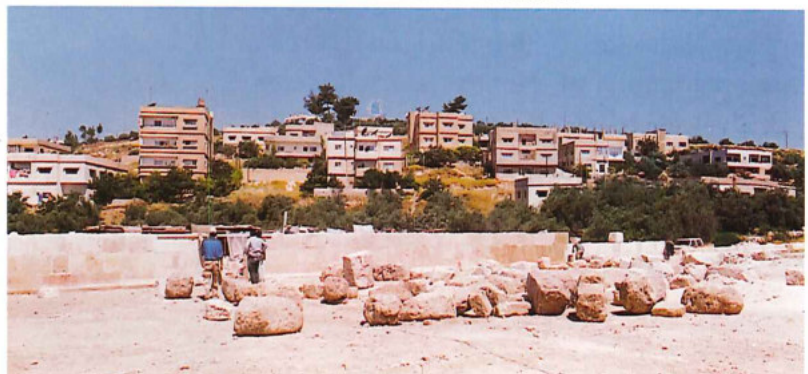
The western wall after restoration
