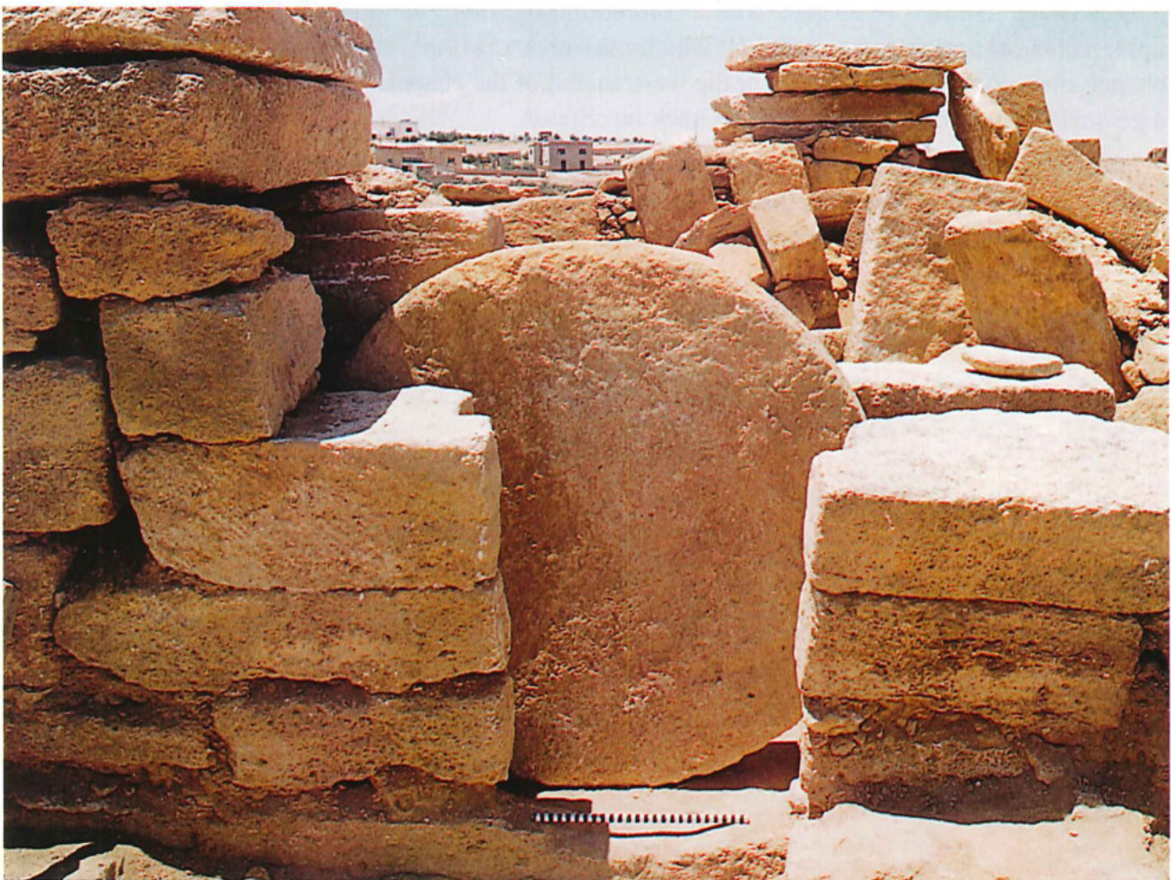
The doorway in the eastern wall, which has a stone disc-shaped door
