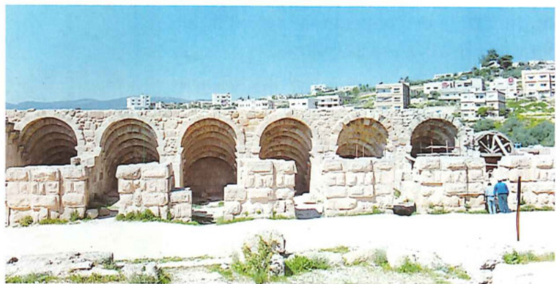
The vaulted rooms after restoration
