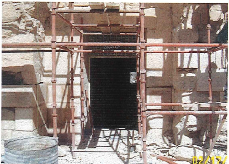
The entrance façade during the restoration
