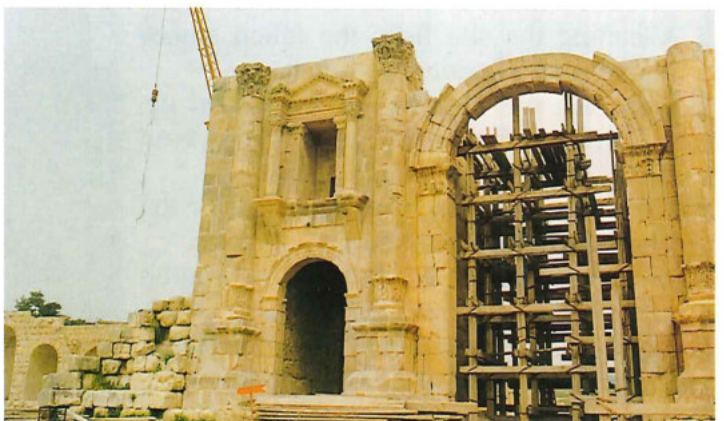
The southern façade after restoration
