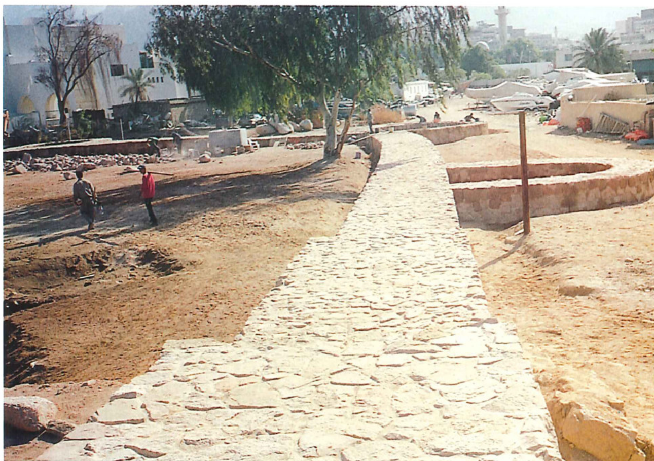
The city wall after the restoration
