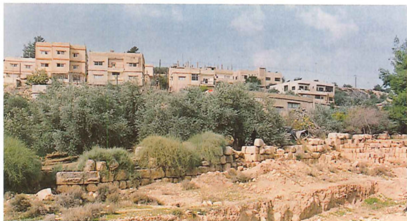
The western wall before restoration
