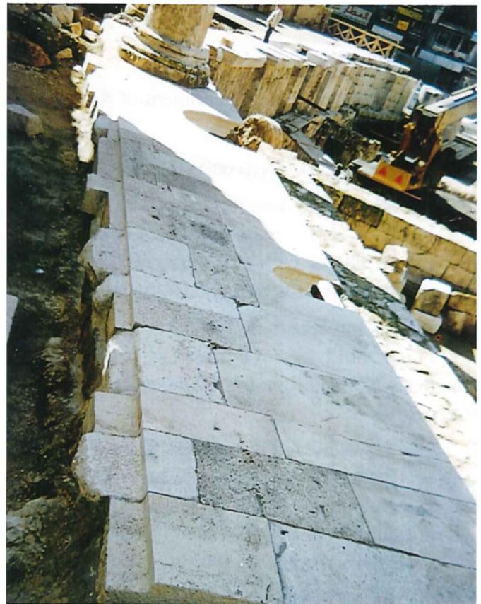
Part of the cornice of the first level
