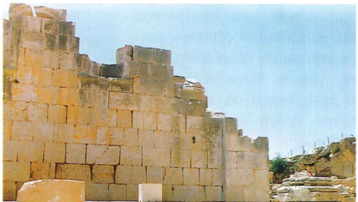
The western façade of Zeus temple after restoration
