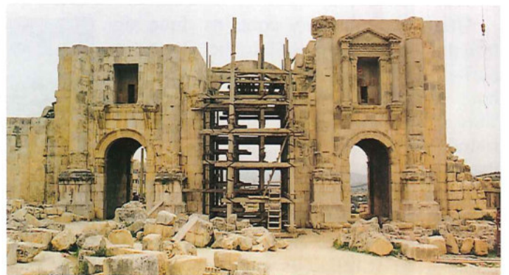
The northern façade after restoration
