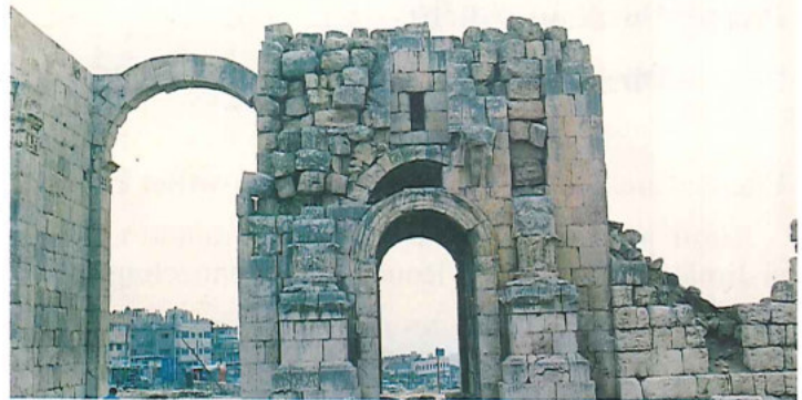
The northern façade before restoration
