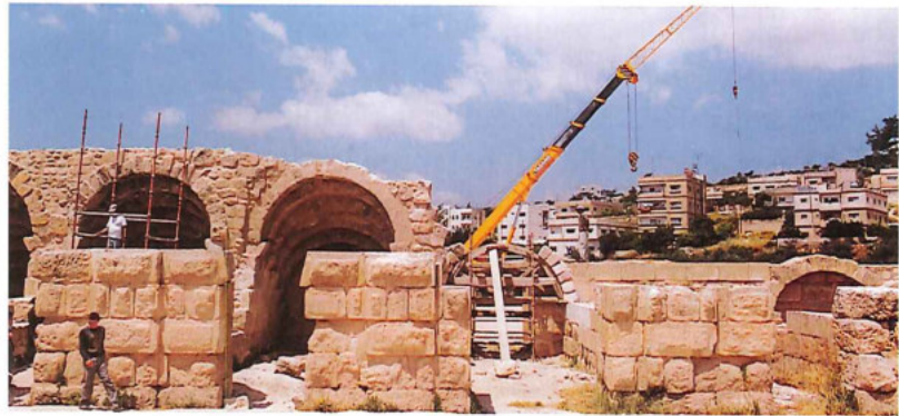
The vaulted rooms during restoration
