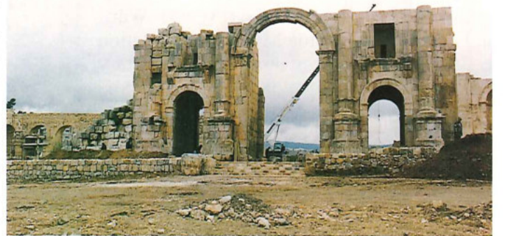
The southern façade before restoration
