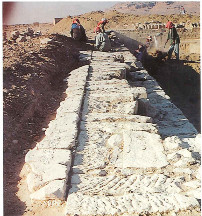
The restoration works at the water reservoir
