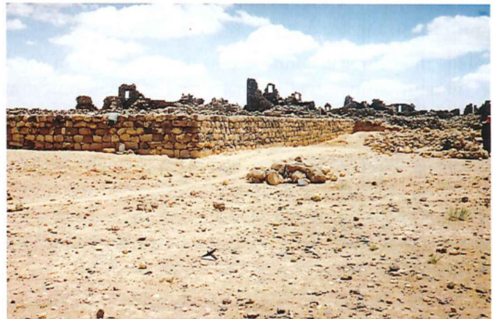
The city wall after the restoration
