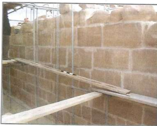
Consolidation and reconstruction work of the Temple
