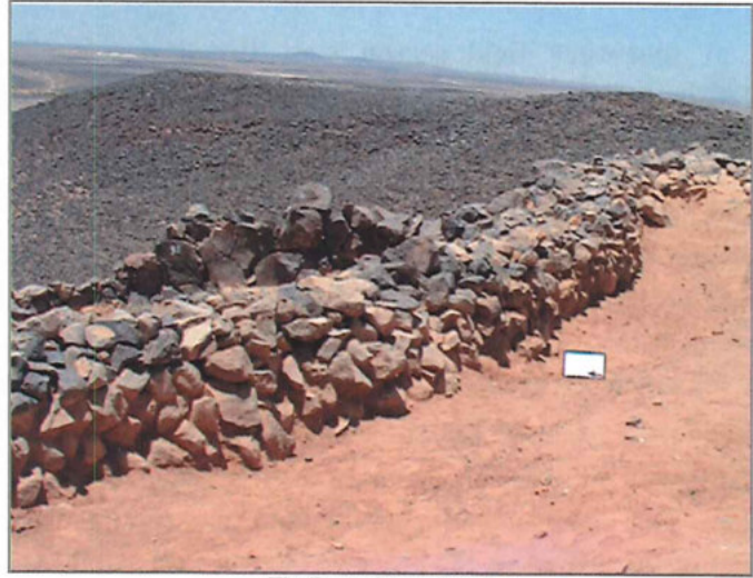
The Dam after restoration
