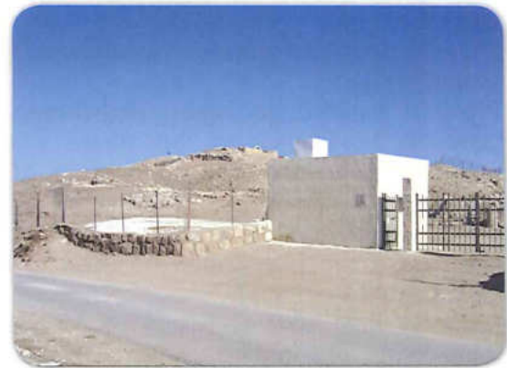
Fig.9 : General view of the new gate
