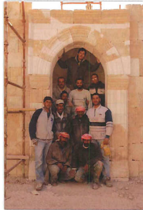
Restoration work : al - mihrab
