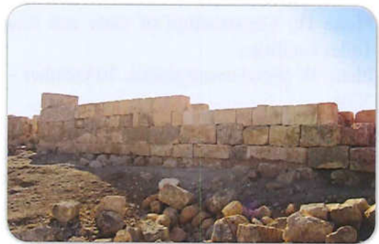
Fig.5 : The Northern wall after restoration
