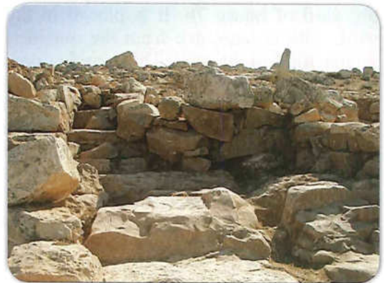
Room in the House 77.
