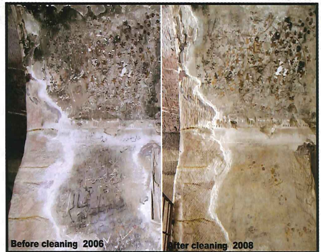
Biclinium 849 vault and wall overview before and after cleaning
