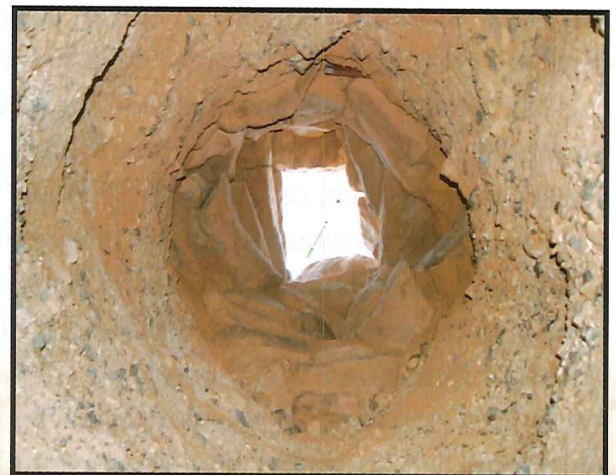
Fig. 2: Qublan Bani Murra: Corbelled masonry of well D15 from inside the well. (photo: H.G.K. Gebel)
