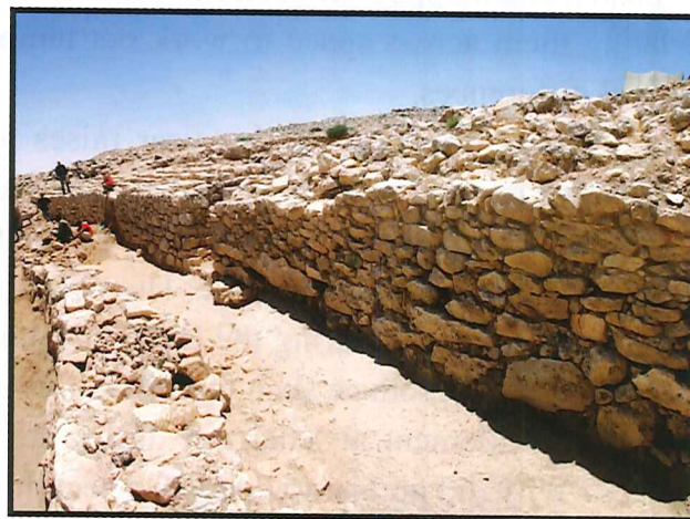
Fig. 1: Area B North. Restoration work at Wall W.155, from west.
