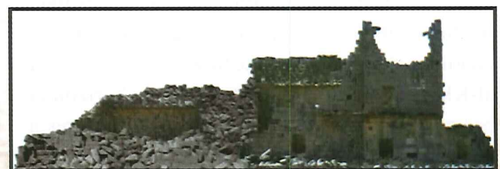
Umm al-Jimal "Barracks". Internal elevation
