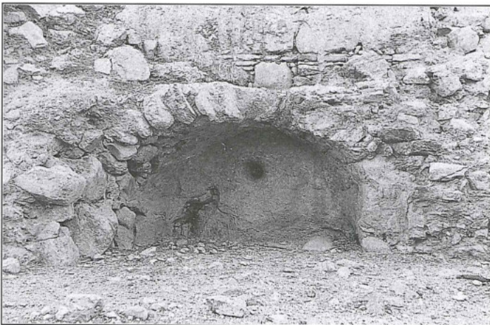
3. Water outlet at the base of the penstock tower from which the water exits under pressure onto the mill-wheel.
