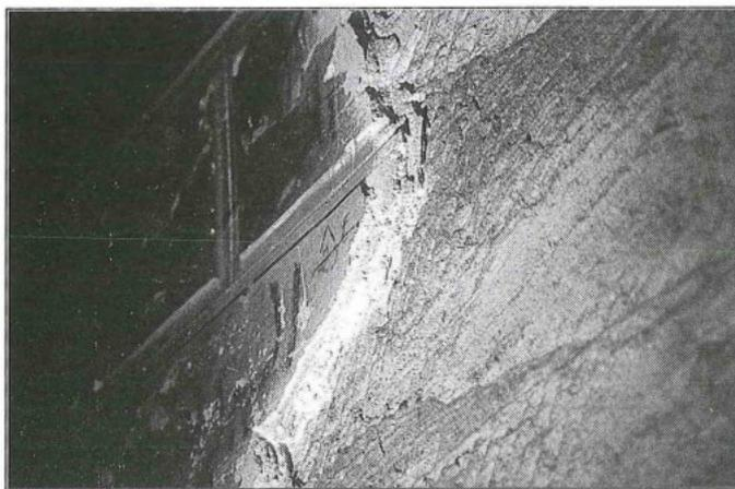
2. Petra frescoes. The triple layer of mortar and the layer of "coating" are visible.
