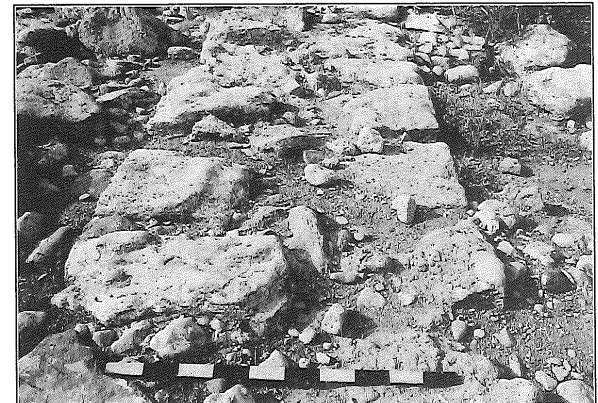
15. Construction of a wall of harbour Zara 21.
