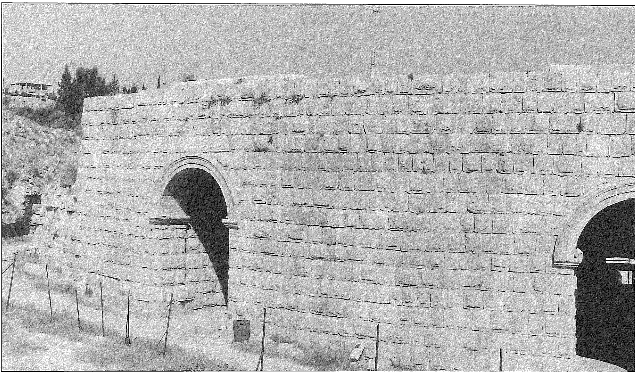
3. Back of the cavea of the South Theatre at Jarash showing the outer wall and the passage behind (173.25A).
