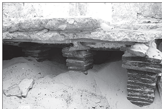
8. Cross-section of hypocaust in tepidarium (Th. Fournet).
