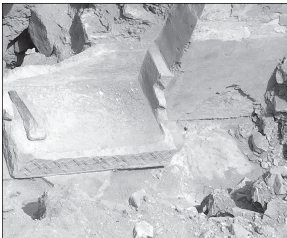
12. Basin in the hot room/ jūwwānī before its destruction by a bulldozer (©Mission Dusaq 2009/ R. Elter).
