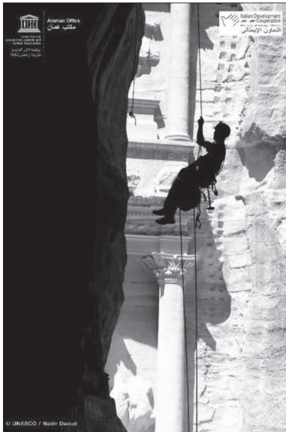
2. Landslide risk mitigation works, © UNESCO.
