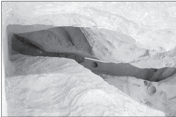
11. View from the top of the main dam down into the outflow channel at the bottom of the retention basin (Photo U. Bellwald).
