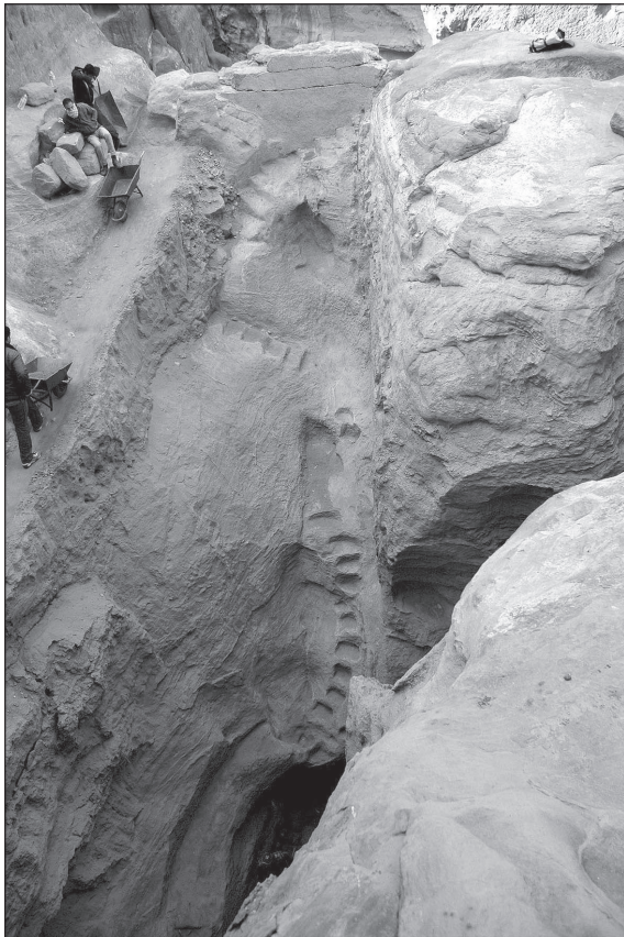
13. View from East onto the Western dam and the maintenance stairs leading down into the retention basin (Photo U. Bellwald).
