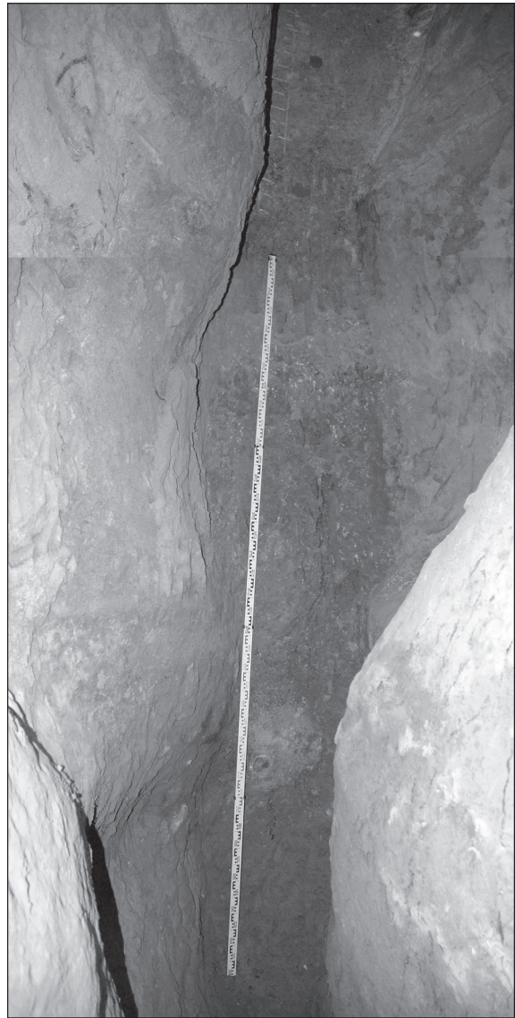
9. View onto the lower part of the upstream face of the main dam with the outflow valve (Photo U. Bellwald).
