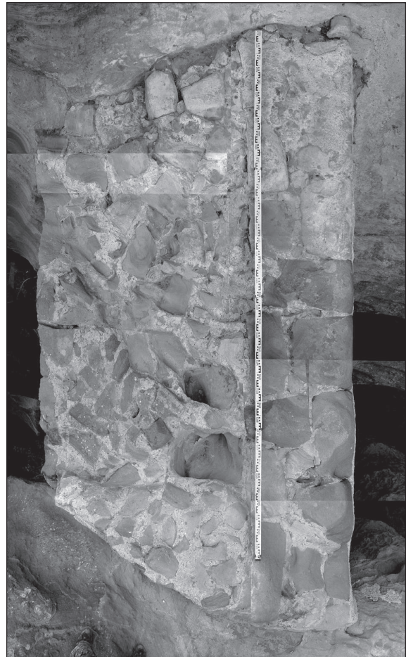
15. View onto the crest of dam nr. 3, assembly of orthogonal photo shoots. The illustration shows well the double sided masonry of the first dam (bottom) and its downstream extension (top) (Photo U. Bellwald).
