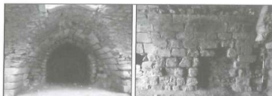
8. CF8: vaulted niche and masonry techniques (Type 3).
