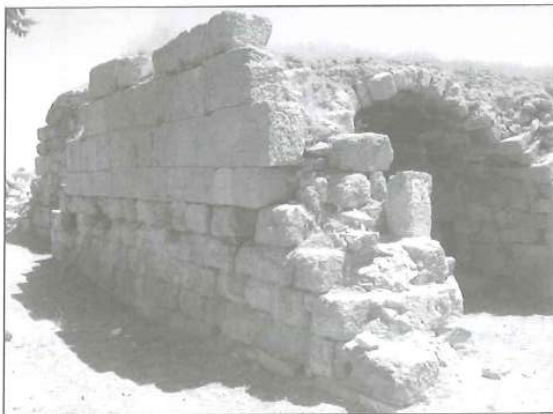
2. Qaṣṭal al-Balqā'. Umayyad wall from the 'Syrian bayt ' to the north of the entrance block/vestibule (facing the court corridor), which presents two different building techniques corresponding to two consecutive building phases (both datable to the Umayyad period). The vault seen to the right, dates from Ayyubid-Mamluk period; it is built within the width of the Umayyad room, and rests on its own walls which double the Umayyad ones (see FIG. 3).
