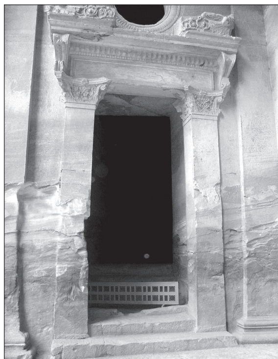
3. View at the doorway in the southern wall of the entrance hall of al-Khaznah, showing the heavy erosion of the sandstone, reaching almost half of its height. This erosion is due to the crystallization of salts during the evaporation of the rising ground humidity in the void of the stone structure in the warm seasons (Photo U. Bellwald).
