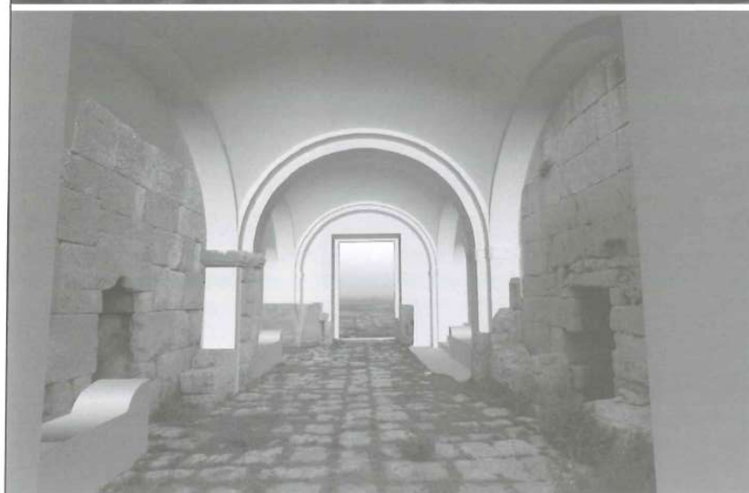
19. Qasṭal al-Balqā'. Umayyad qaṣr. Entrance vestibule. Reconstruction hypothesis. 19a. Present condition of the remaining elements. 19b. Composite view with the infographic reconstruction of the two sail vaults (Reconstruction hypothesis by I. Arce; infographic: I. Moscoso).
