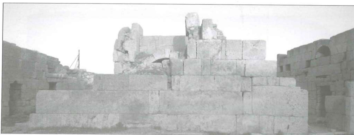
7. Qaṣṭal al-Balqā'. Wall facing the court (corresponding to the second Umayyad phase). Notice the presence of huge ashlars incorporated in its masonry. Behind this wall can be seen the entrance vestibule (to the left), the south flight of stairs (centre), and the 'incomplete' south Syrian bayt (right).
