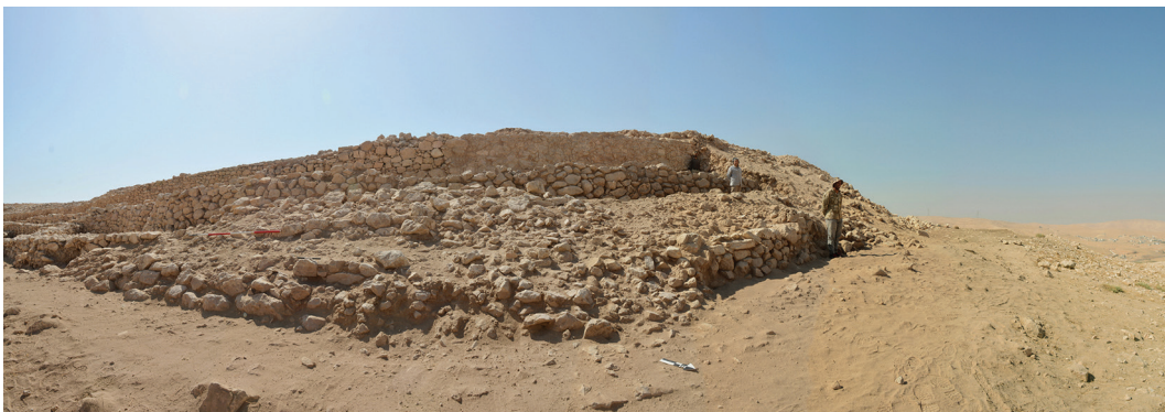
7. View of the northern face of Exterior Wall W.827 with the EB IVB Embankment which concealed the EB III collapsed walls, seen from the north-east.
