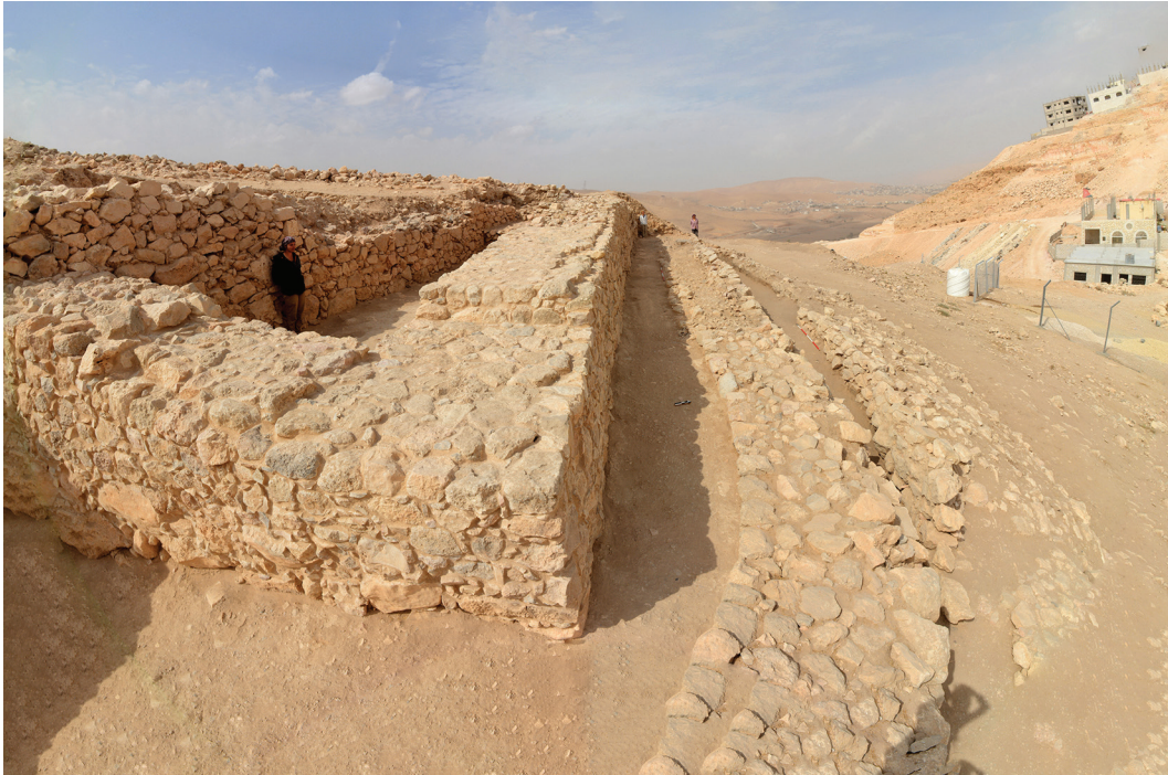
4. View of Northern Bastion T.830 and Gate L.860 inside it, seen from the east (after the restoration of the outer wall of the Bastion).
