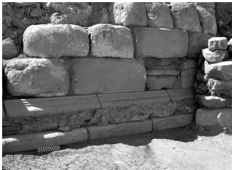
9. Pipeline B in situ set into the decorative molding along the base of the pool's façade wall, adjacent to the west Staircase, and sealed in place with mortar and pottery sherds.
