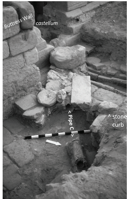
10. Pipeline C in situ with other components of a makeshift catchment basin that reused features (the castellum, stone conduits, and modified column drum) of the earlier garden site.
