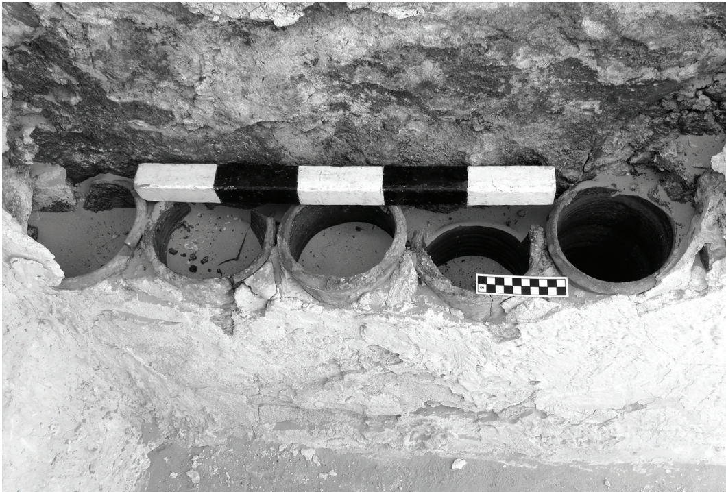
5. Close-up photograph of cylindrical heating pipes in situ in southeast corner of the tepidarium (R. Darby).
