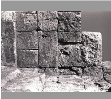
8. Blocked sally port.
