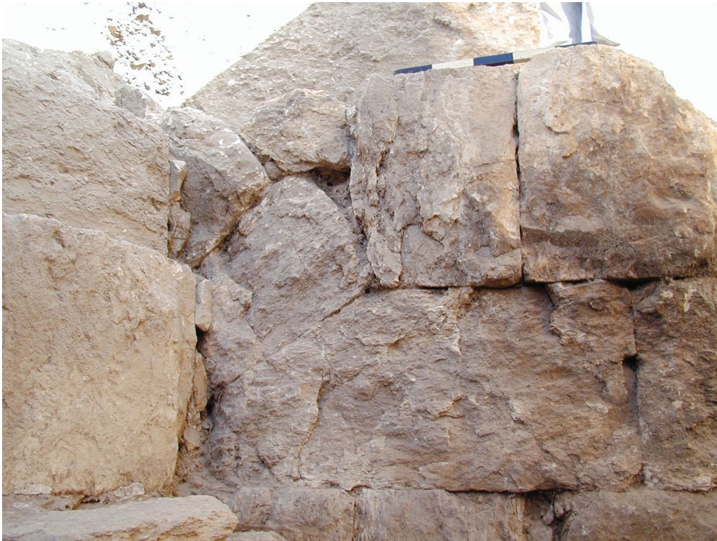
3. Approach of a segmental arch over Gate 3.
