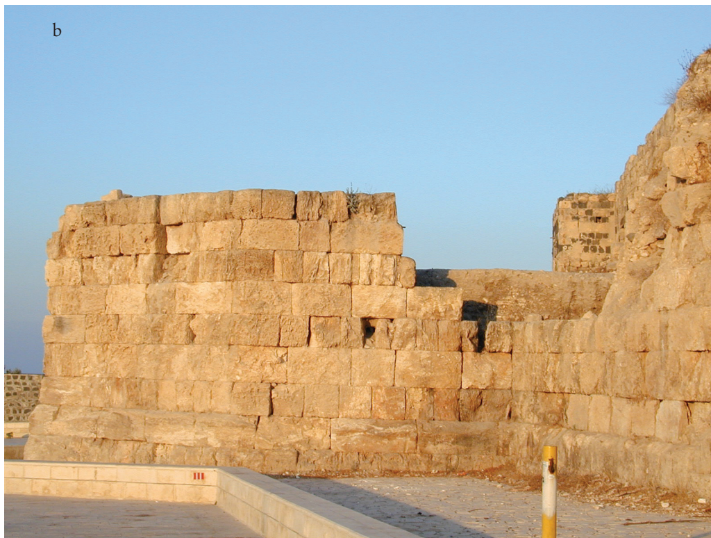
7. Tower 3 from the east.
