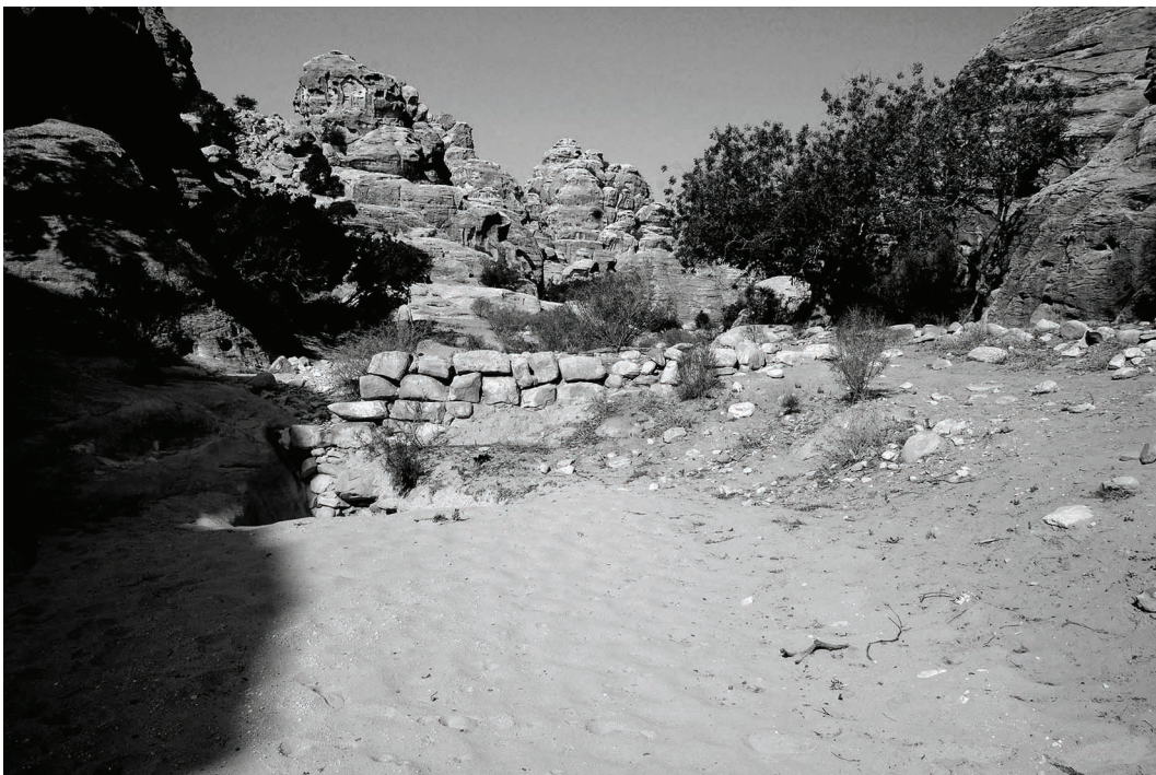
13–14. View of the downstream face of two well preserved average wādī barriers in the central section of Wādī ‘Agalāt. The photographs show that the abutments of the construction touch the bottom of the cliffs. The dry masonry of these wide barriers with limited height has been erected with the same well-dressed ashlar blocks as in the main and major wādī barriers (U. Bellwald).
