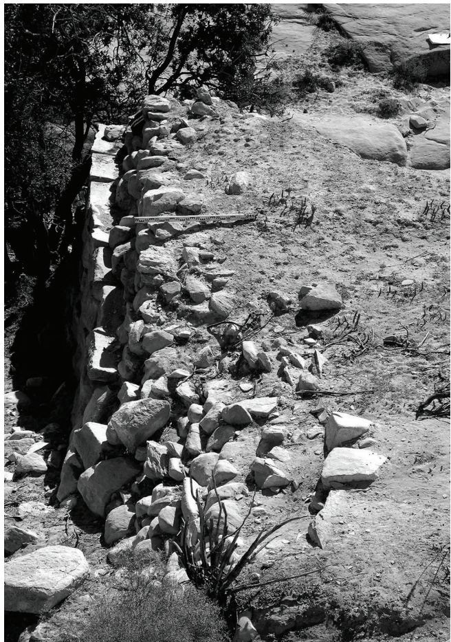
9. View of the well preserved northern section of the downstream face of the main wādī barriers at the northern foot of the rock outcrop bearing the ruins of the farmstead. The frontal view shows well the typical construction method of wādī barriers, well-dressed ashlar blocks set up as dry masonry without mortar (U. Bellwald).
