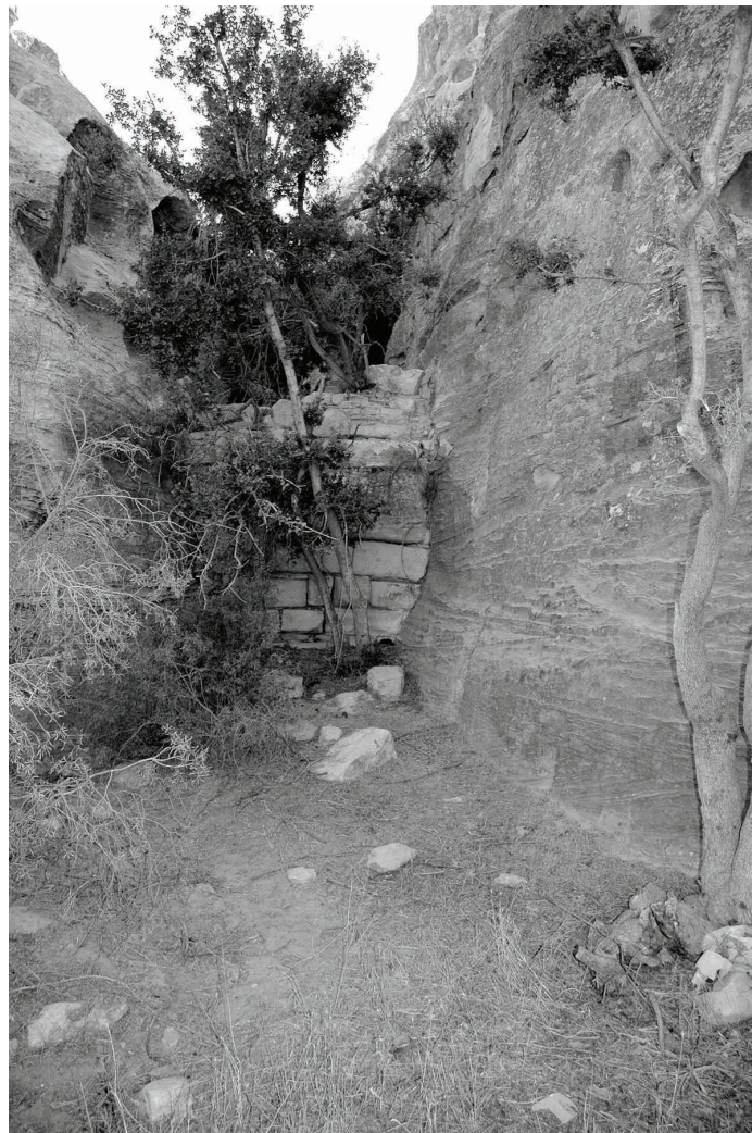
23. The retention dam for storing runoff water south of the eastern wine press. It closes a long and narrow fault running parallel to Sīq al Bārid (U. Bellwald).
