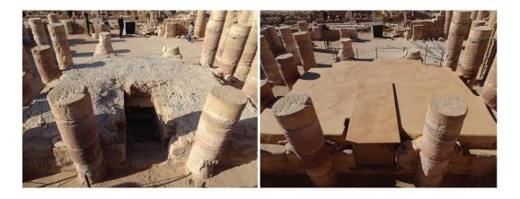
20. Before and after the application of a protective mortar capping on the Cella podium in 2017. Photos by Franco Sciorilli.
