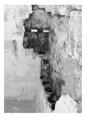
these cylindrical pipes were primarily found in the *tepidarium*, where they comprise the near entirety of the wallheating system (FIGS. 4–5). Several of these tubes were also found in the *caldarium*. While the installation of these pipes against the wall in columns allowed for the vertical flow of hot air from the hypocaust, the lack of lateral vents like those on rectangular *tubuli* prevented
