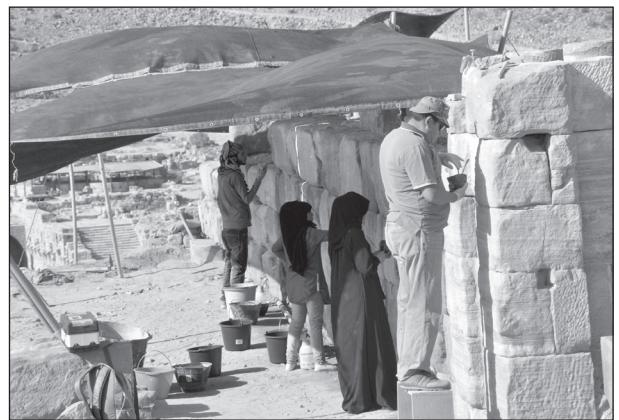
6. Conservation training in action. Mortaring of the east wall of the cella in 2016 (photo: USAID SCHEP, ACOR).
