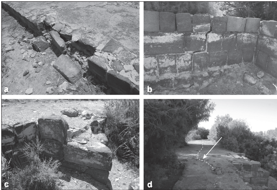
20. Damage on the wall of the reservoir-enclosure located inside the reserve, on the tourist track (zone II): a) lifting of facing blocks; b) transverse cracking in the wall; c) falling of blocks; d) longitudinal crack on Massif C (AASRP 2015).
