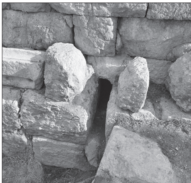
11. Southern pteroma. The inlet to the cistern through the slot in the foundation of the south wall of the cella (photo: M. Brizzi).
