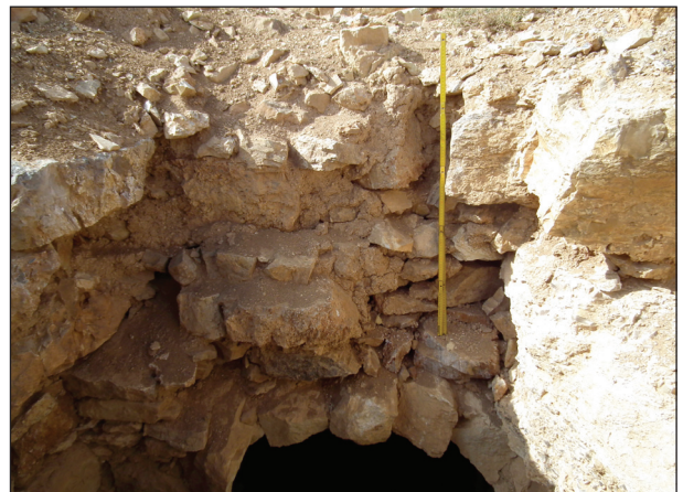
8. Section of roofing of PHTP Tomb 2 (facing west) (L. Wadeson).
