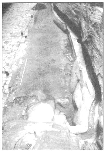
4. The gravity flow channel of the as-Sīq aqueduct, built mid first century AD. The section shown includes a settling tank (top right).
