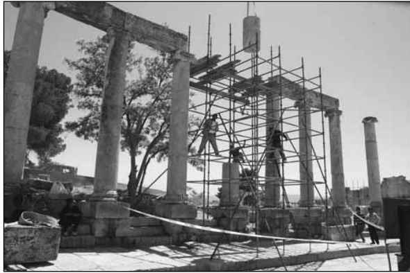
2. Oval Plaza: the disassembled and anastylosis of column 31.
