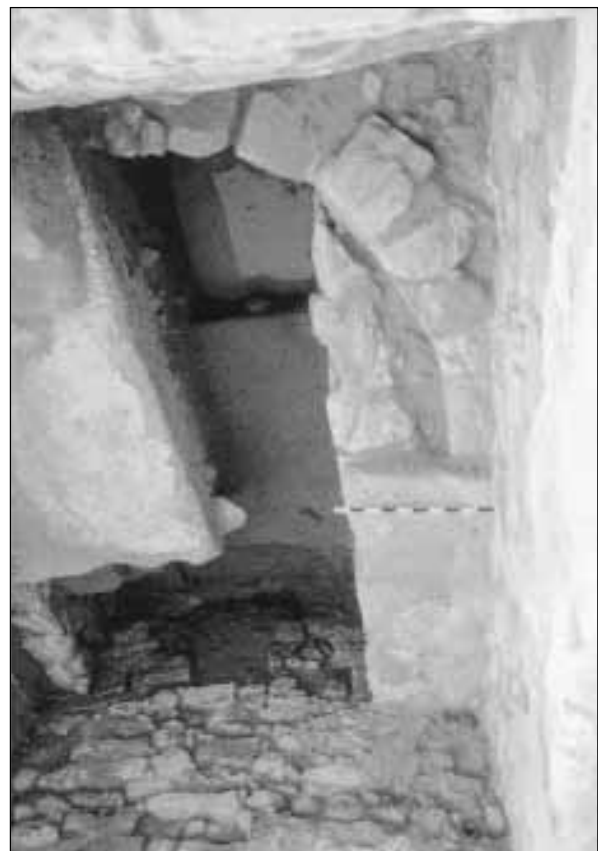
2. The square tower, showing the original U-shaped tower, door through the city wall, and water table.
