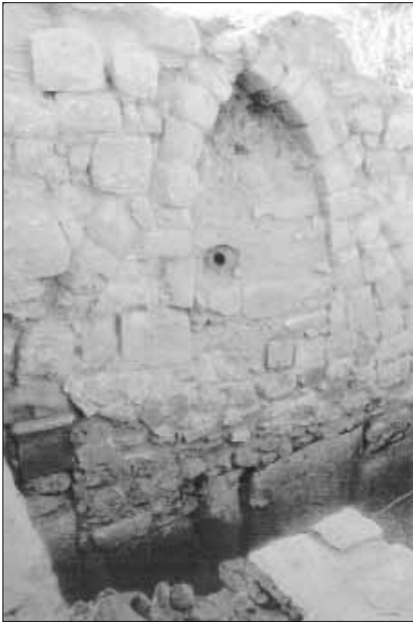
12. Exterior of the Egyptian Gate, showing original wide gate with arch, early blockage of half with column, complete blocking preceding insertion of narrow doorway and pointed arch.
