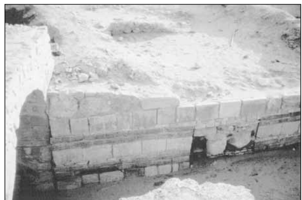
11. Building with ablaq and blocked doorway, east of inner arch (E8d, E9c).
