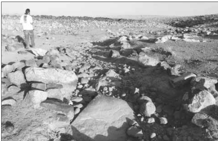
5. Beginning of ancient Umm al-Jimāl water supply channel at its diversion point on the Wādī az-Za'atari approximately 5km NE of Umm al-Jimāl. The channel, still functional, is in foreground, the wadi in the background. (15 January 2010. Photo by Bert de Vries).
