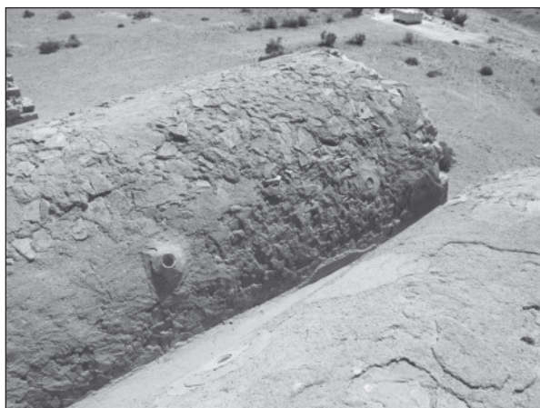
6. Condition of the extrados of the vaults (before intervention).
