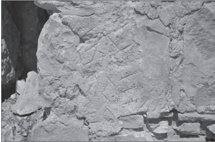
4. Original mortar found on the exterior of the monument.
