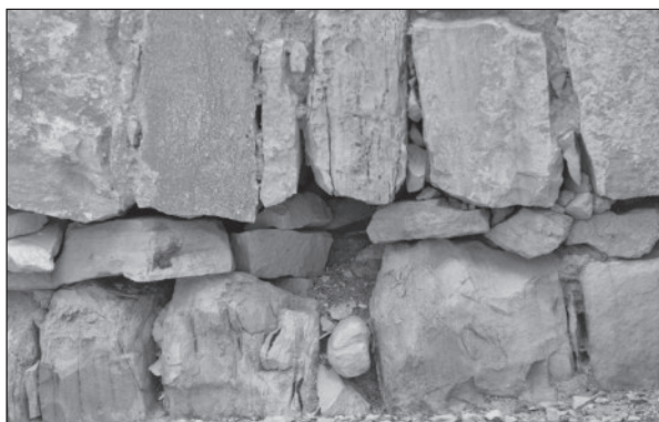
5. Mortar loss at the base of the walls (before intervention).
