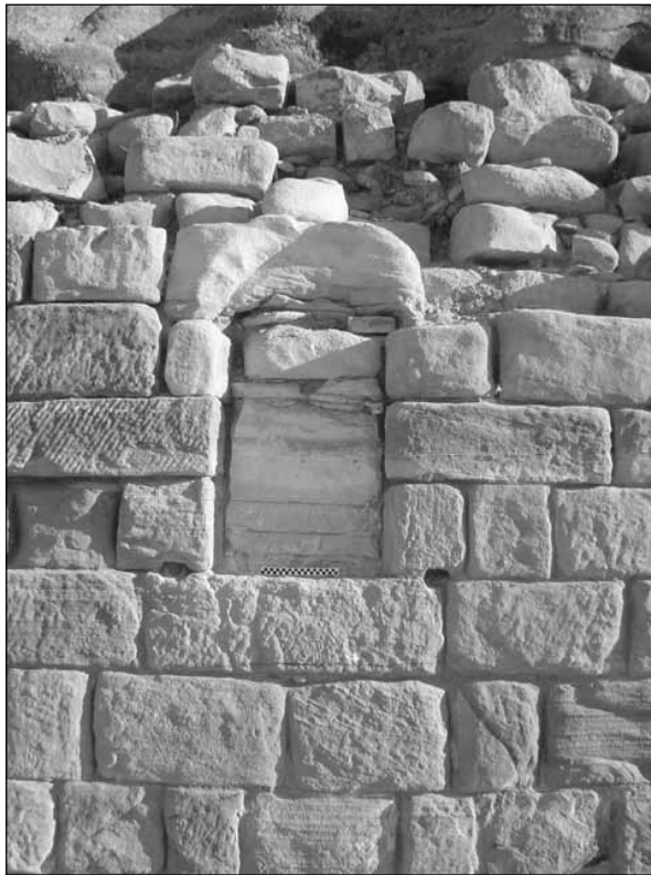
4. Central niche ( nefesh ) in the south wall façade.
