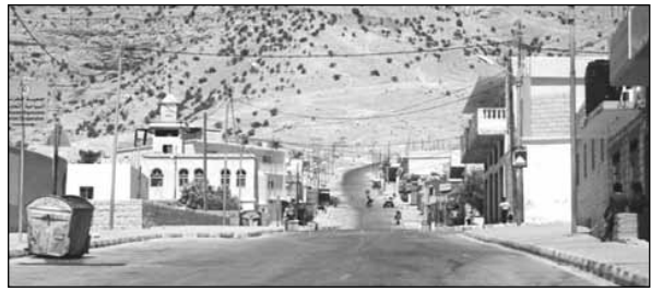
5. A view looking up the main street of Umm Şayhūn. Only paved in the mid-1990s, the road now represents the main artery for commerce, transportation and utilities (e.g. water, electricity) in Umm Şayhūn and Bayda (photograph by Paradise).
