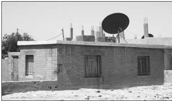
3. An original single storey, simple cement block house built in the 1980s (photograph by Paradise 2007).
