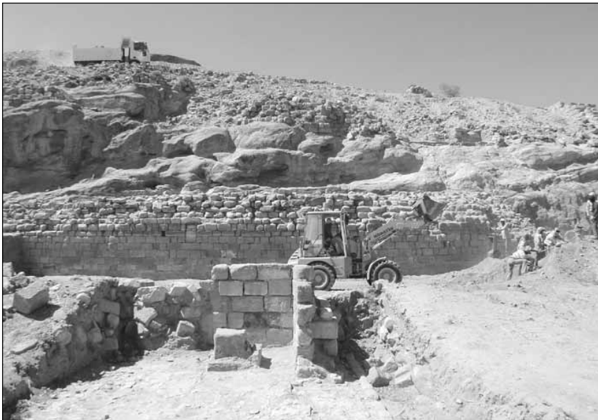
3. Removal of excavated overburden from the site with a backhoe and dump truck; island-pavilion in foreground.
