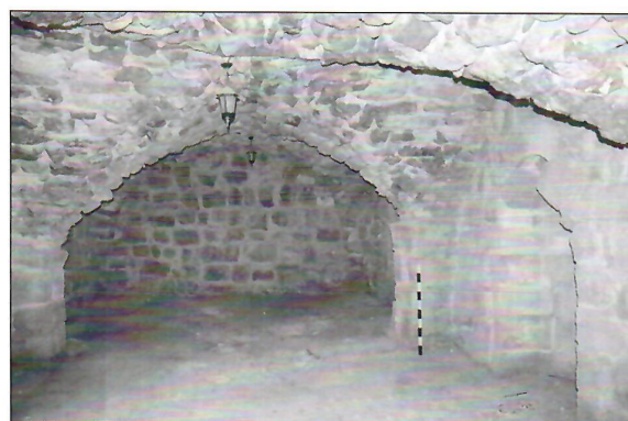
21. Interior of Maqām Shaykh Khalīl - note barrel vaults supported on engaged piers, mihrāb to right.
