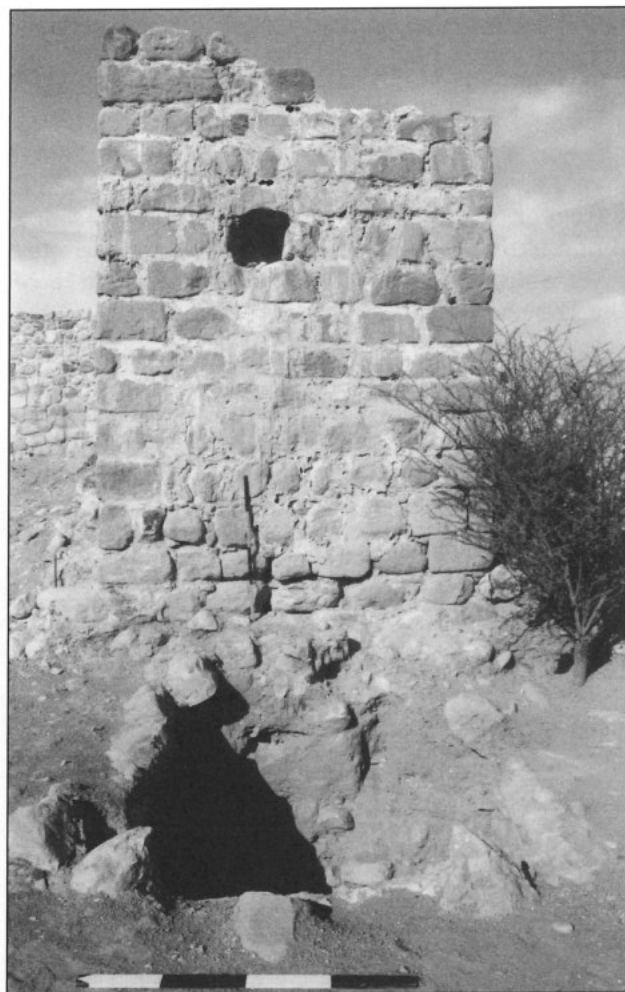
12. Vertical penstock of western mill at Ṭawāḥin as-Sukkar (photo: K. D. Politis).
