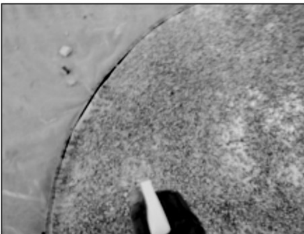
22. Before applying the new mortar to the fibreglass, both fibreglass and tesserae were wetted by spraying water.
