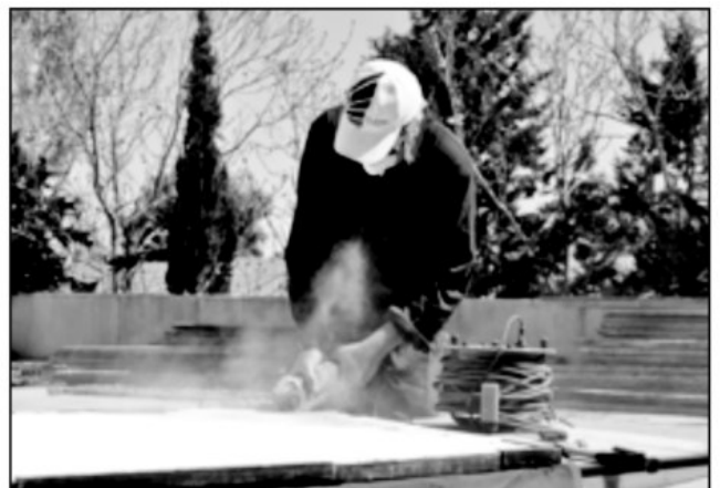
13. The process of removing the mortar started with the use of a grinder to create small squares.
