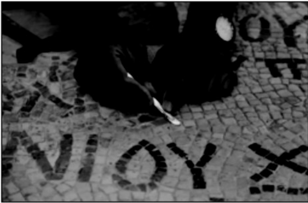
26. The mosaic was left to dry and then rinsed with water. A rough brush was used to remove glue and calcination; the remnants of the old glue used in the first restoration were removed mechanically using a scalpel.
