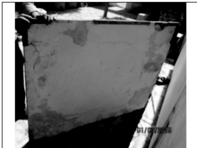
4. The restoration team placed a metal mesh within the new mortar, which can lead to rust forming on the surface of the mosaic.
