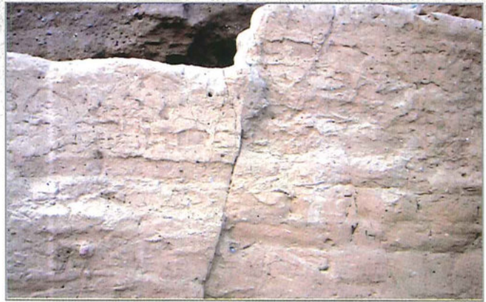
The Byzantine church showing rupture caused by earthquakes
