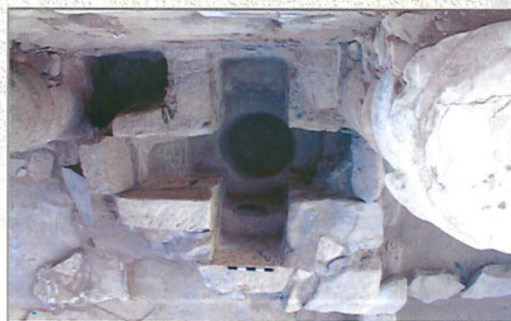
Masonry-built cruciform font
