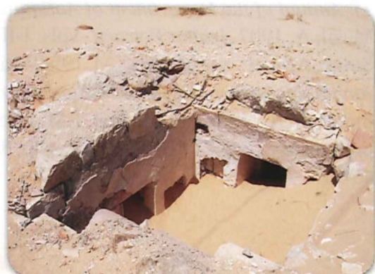
Fig.3: Concrete birka with reused ashlar masonry/, Modern
