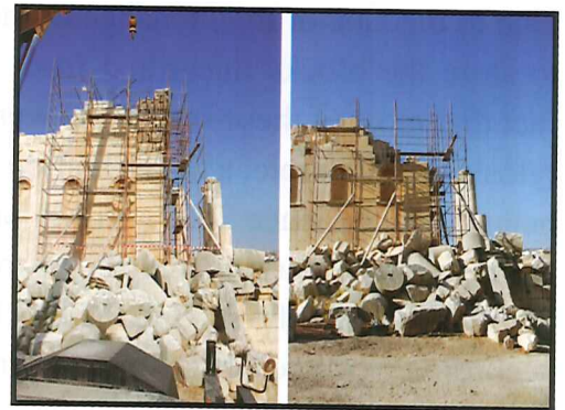
Fig. 4: Restoration of the South-Eastern Corner of the Cella: Before and After Dismantling (Photo S. Desoutter © IFPO 2008).
