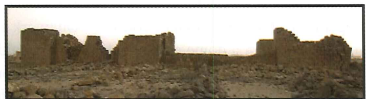
Dayr al-kahif. North walls. External elevation
