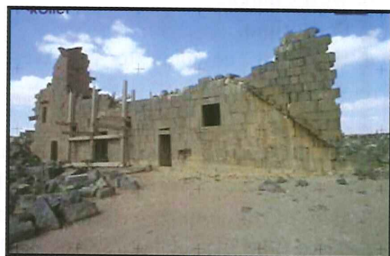
Image from the "Praetorium" taken with a metric camera for Photogrammetric recording
