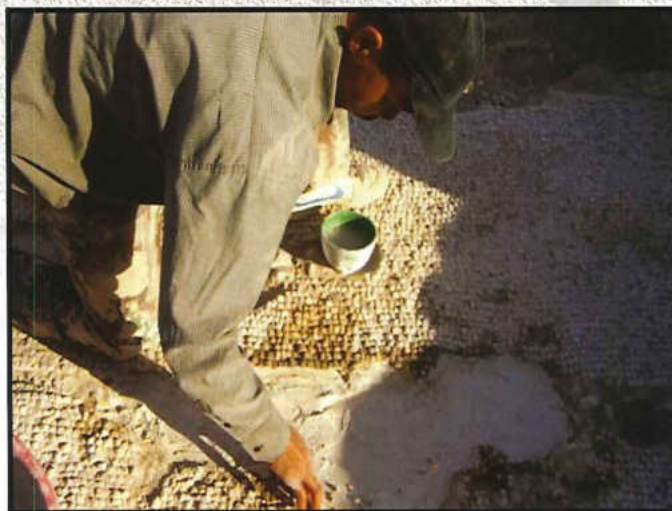
Fig. 6: Fill damaged area with mixture
